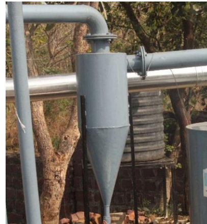
Figure 9: cyclone Separator
